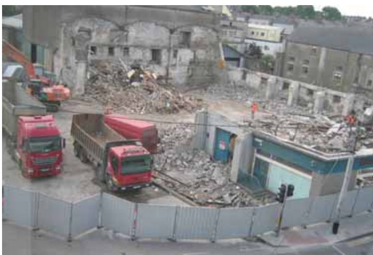
Demolition and preparation of site for screening unit in Cork
