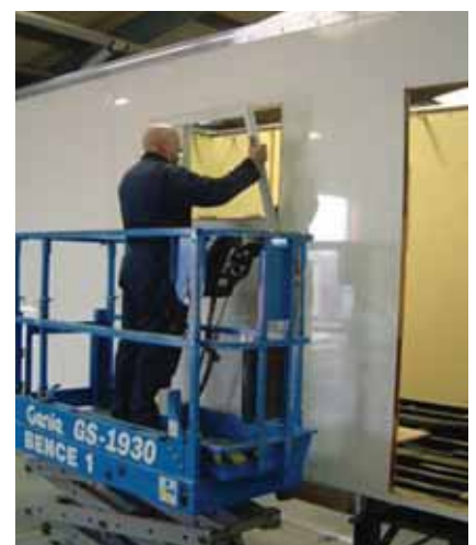
Screening mobile unit in construction
