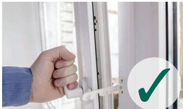
Window restrictors prevent a child from opening windows where they can fall
