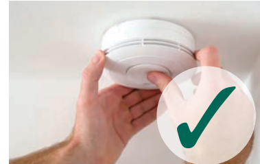
Check the smoke alarm
